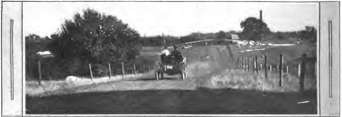
Where the New Dirt Road Was Made Connecting Burman Avenue and the Boulevard
